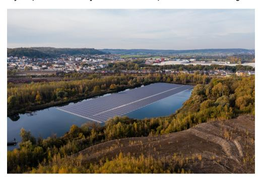
The floating solar farm has been installed on a former cooling pond belonging to ArcelorMittal Differdange, and consists of 25,000m2 of solar panels, with a surface area of 5.7 hectares. Eventually, the electricity produced will amount to 3 GWh/year and will be able to power nearly 800 local homes, i.e. the annual electricity usage of 3,200 people\*. The electricity produced on the floating solar
